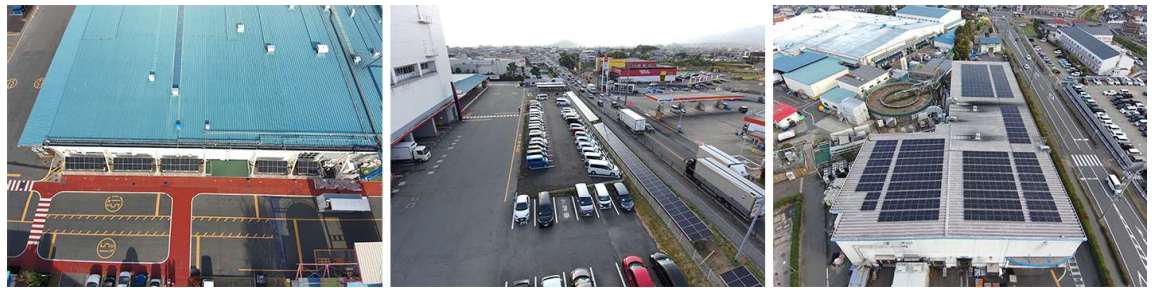
Three solar panel installations on the premises of Tosu Kewpie Co., Ltd.
