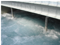
Hollow fiber membrane module unit (air diffusion)
