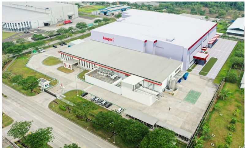
Illustration of the plant with the completed additional lines (PT KEWPIE INDONESIA’s head office plant)
